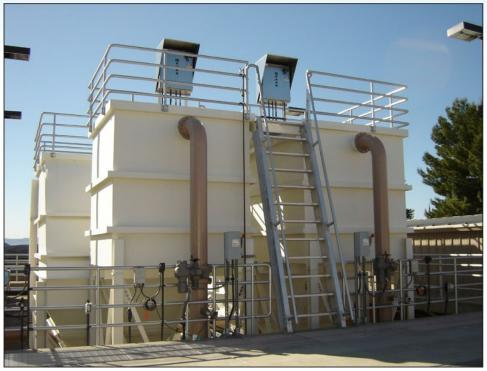
With the help of WesTech's SuperSettler inclined plate clarifiers, CLWA was able to increase total plant capacity while consistently meeting turbidity requirements.
