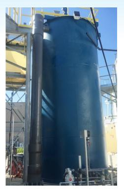
reaction tank 1 where lime addition was used to adjust pH. Water flowed via gravity through two more reaction tanks where ferric chloride and organosulfide were added to precipitate the metal hydroxides. In addition, polymer was added for flocculation. From there, the water was sent to a clarifier to settle and remove solids. The water was then fed into the second half of the treatment train, which consisted of a sand filter followed by a biological treatment system for selenium reduction.
