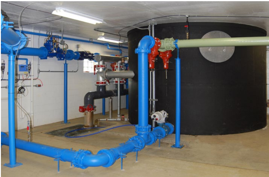
The visible section of the AERALATER is covered with insulation to minimize condensation.
