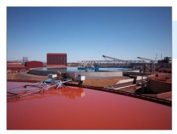
For high-tonnage / high-torque applications, a WesTech Titan  $^{\text{TM}}$  traction thickener can be used as an ideal, economical alternative to conventional center-driven, high-rate thickeners.
