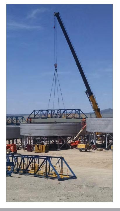
Field erection of process tanks, with the installation of clarifier/thickener internals by WesTech, ensures that the unit will fit together and function as intended. WesTech has the experience, engineering, and fabrication resources to make sure your project comes in within budget and on time.
