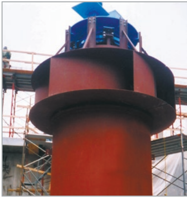
Centrifugal Impeller Pump and Draft Tube
