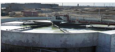
Rectangular tanks are easier to install while circular DAF designs require less maintenance
