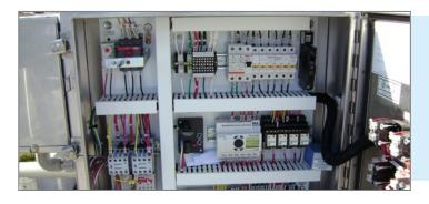
WesTech operates a full-service electrical controls shop that builds custom machine control centers for WesTech process equipment and for other controls applications. From simple control boxes to large control centers utilizing the latest in programmable logic, interactive touch screens and broadly versatile VFD systems, WesTech builds them all under the quality guidelines mandated by ISO 9001 certification.
