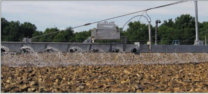
Controlling the dosing rate of the trickling filter is the key feature of the HydroDoc. WesTech has successfully provided hundreds of distributors that offer these process advantages.
