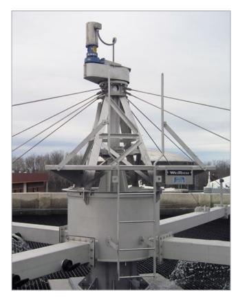
The average U.S. trickling filter distributor should be slowed to 5-10 percent of its current rotational rate.
