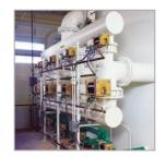
All AERALATER units are provided with a control cabinet for operation of the well pumps and high-service pumps based on the water level in the storage tank. The panel also operates the aerator blower and chemical feeders, based on the operation of the well pumps. When desired, control systems are provided to automatically step the AERALATER through a backwash and return it to service.
