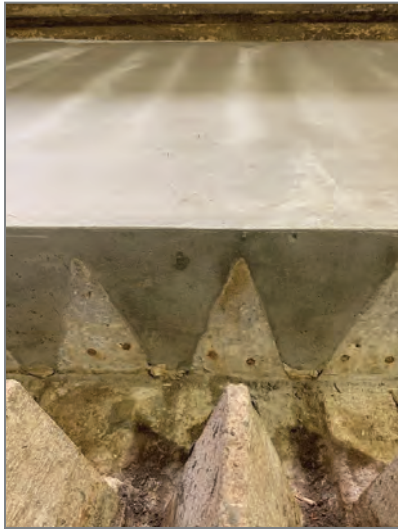
Existing underdrain teepees with concrete fill
