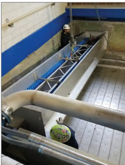
Installing MULTIWASH with LAZERFLO underdrain system
