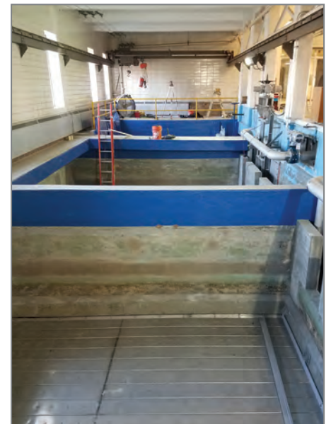
Completed LAZERFLO underdrain
