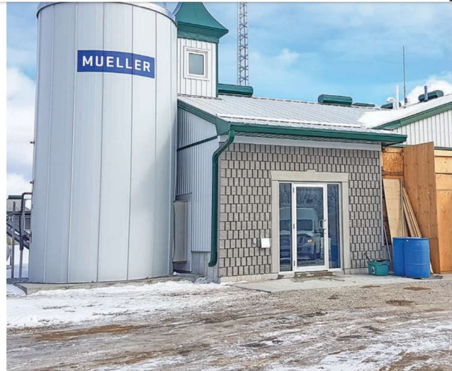
With the milk tower in place on Grootendorst Farms, it holds two days' worth of the farm's milk (38,000 litres) and holds it at a steady 3°C.
