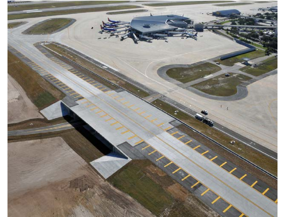
TPA Taxiway B and Bridge
