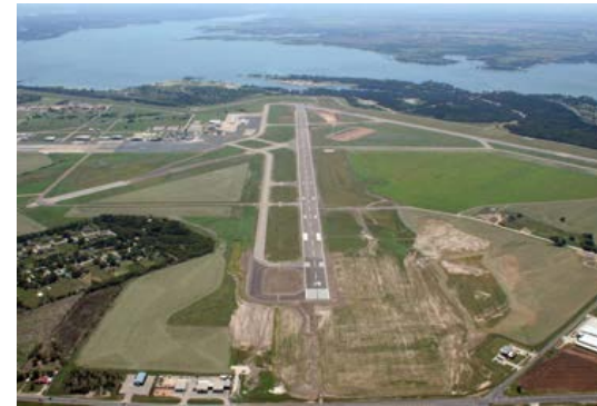
Waco Runway 1-19 Rehabilitation
