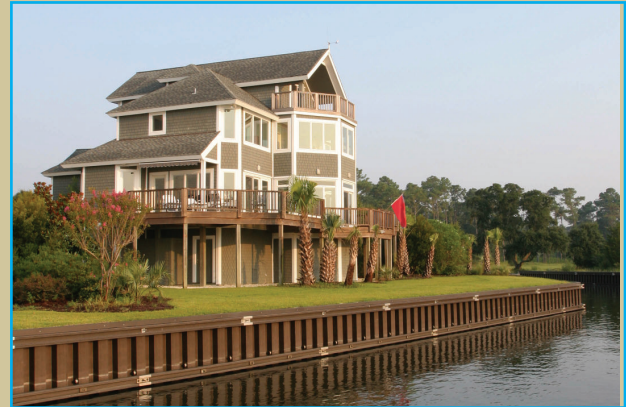
Finished Installation/SuperLoc™ Series 1560, Wales and Top Cap
