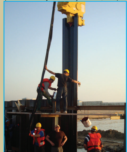
Example of Driving SuperLoc™ Sheet Piles
