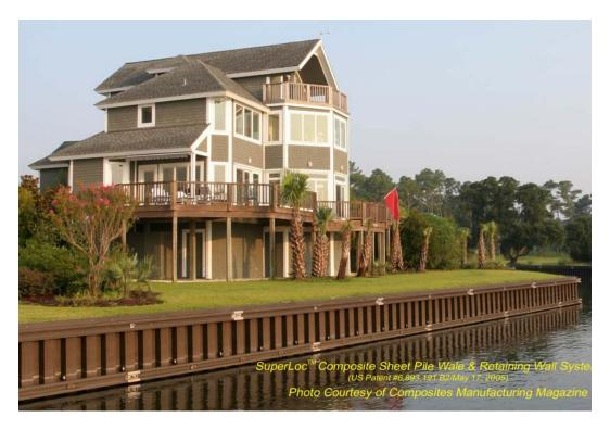
Figure 7.0 Superloc<sup>™</sup> Sheetpile system with the polyurethane cap
