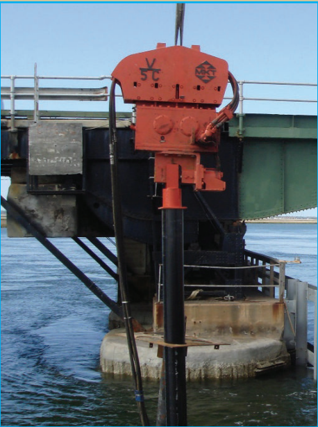
Example of Vibratory Hammer Steel Fabrication
