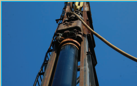
Vulcan 01 Impact Hammer Driving 16" Diameter SUPERPILE
