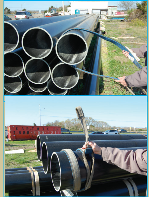
Lift-It® Sling Double Wrapped Around SUPERPILE
