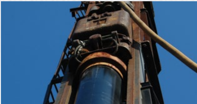
Vulcan 01 Impact Hammer Driving 16" Diameter SUPERPILE®
