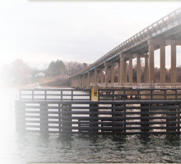
Fender Rehabilitation Route 3 Over Piankatank River, Virginia
