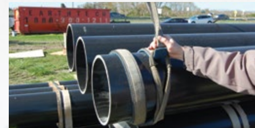
Lift-It® Sling Double Wrapped Around SUPERPILE®
