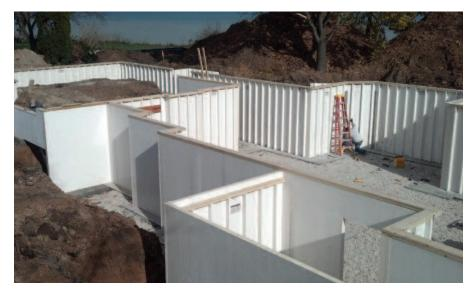
A new foundation-wall system of foam-cored fiberglass panels replaces poured concrete to create warmer, drier, more energy-efficient foundations that reportedly are structurally dependable for the life of the home. On a standard-size dwelling, foundation walls can be erected in less than two hours by crews with standard trade skills and minimal training. The wall system is said to be cost competitive anywhere concrete foundations are installed. (Photo courtesy of Composite Panel Systems, LLC.)
