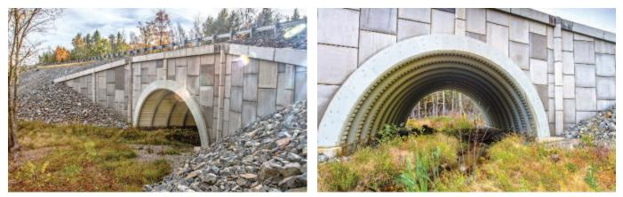
A composites-intensive bridge technology developed by the University of Maine is said to provide a better and faster way to replace a wide variety of concrete and other bridges. The composite bridge uses "inflatable arches"—Portland cement-filled resin-infused textile sleeves that provide a permanent form for concrete—creating an exoskeleton that eliminates the need for rebar and protects concrete from water and environmental damage. (Photos courtesy of University of Maine.)
