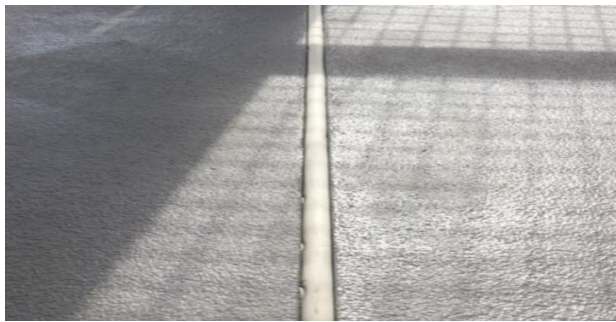
Figure 9 – Colorseal System Installed Between Two Panels
