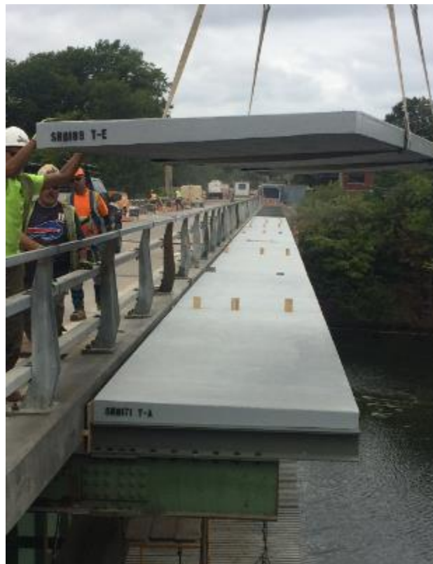
Figure 6 – Wooded shims used to set panel spacing
