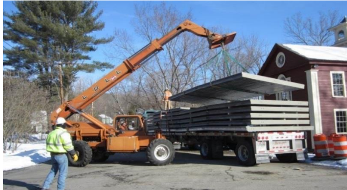
Figure 2 - Typical unloading of truck
