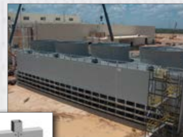
COMPOSITE COOLING TOWERS constructed with custom patented pultruded profiles
