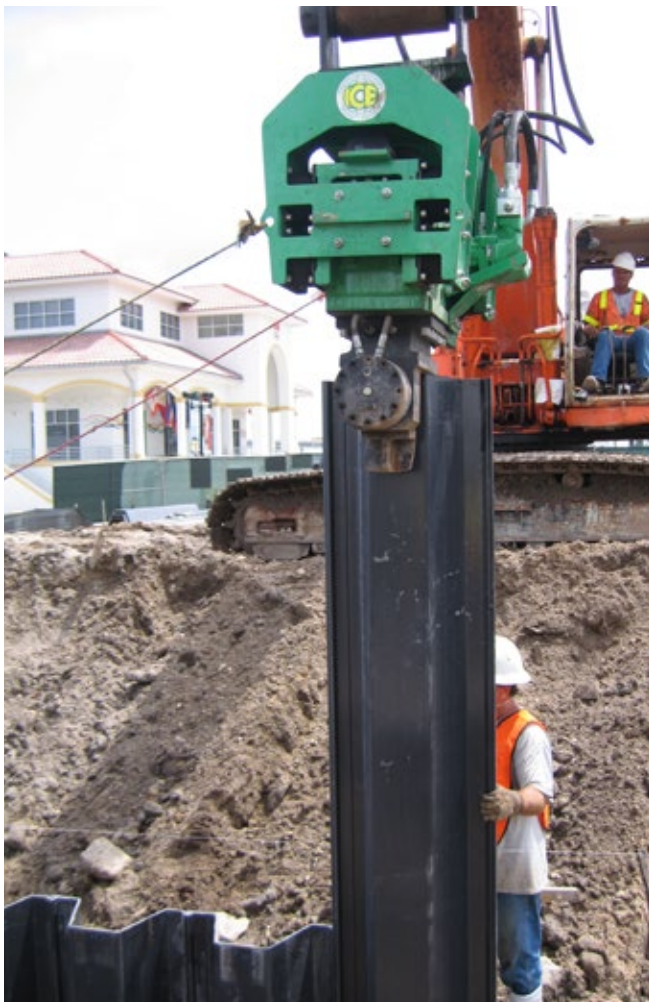
Vibratory Hammer Installation Example
