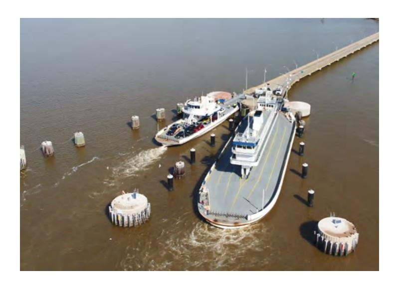
Breasting dolphins also assist in forming buffer zones between vessels and piers or other structures, preventing the vessel from pressing against and damaging a pier structure. Breasting dolphins can also serve as mooring points to restrict longitudinal and/or lateral movement of a moored or docked vessel. Because they serve many functions, breasting dolphins are seen as a cost-efficient way to enhance a berthing safety.
