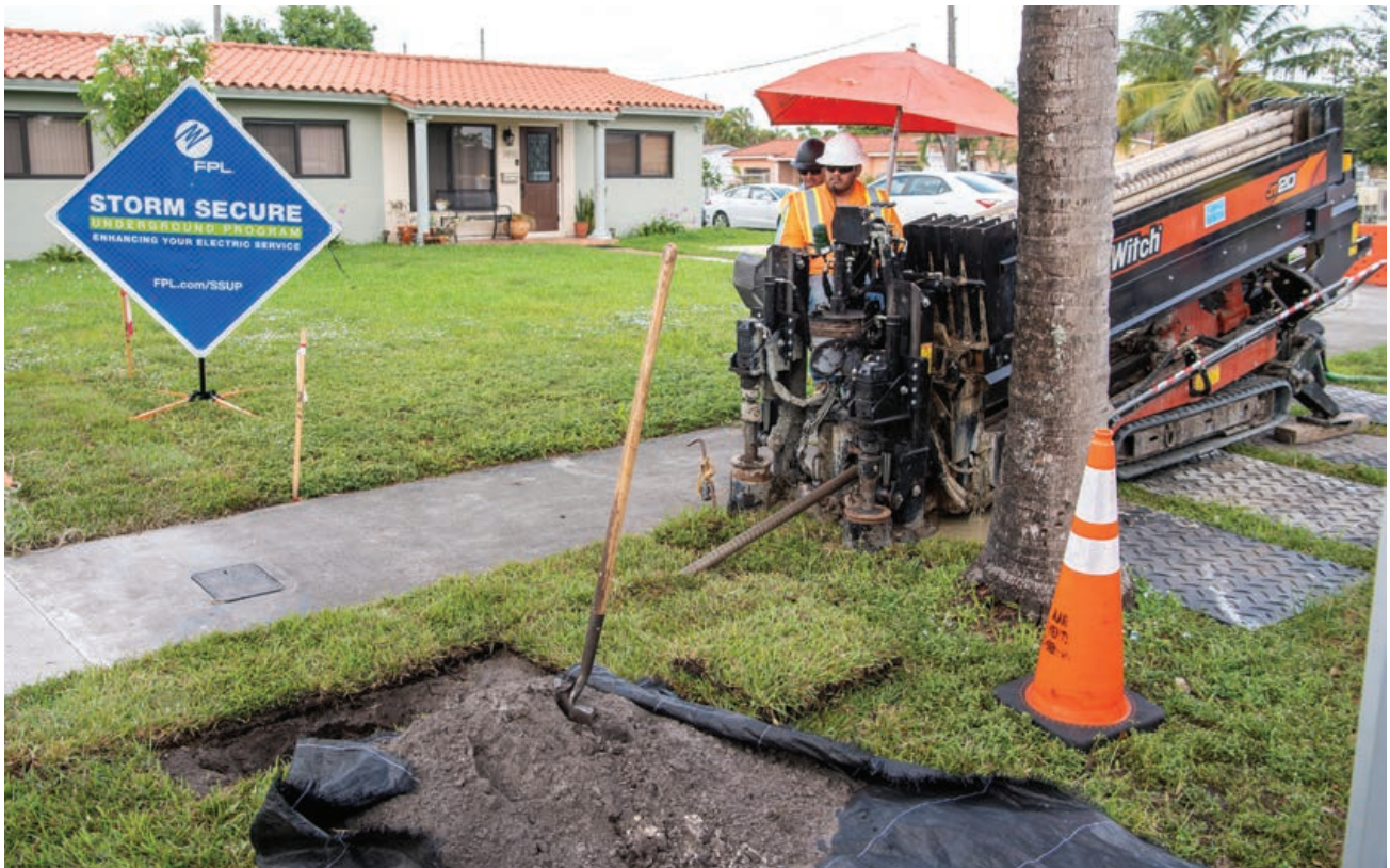
FPL uses directional boring to minimize disruptions when installing underground power lines in its Storm Secure Underground Pilot Program. When complete, FPL restores property to its previous condition. This is in Hialeah.
