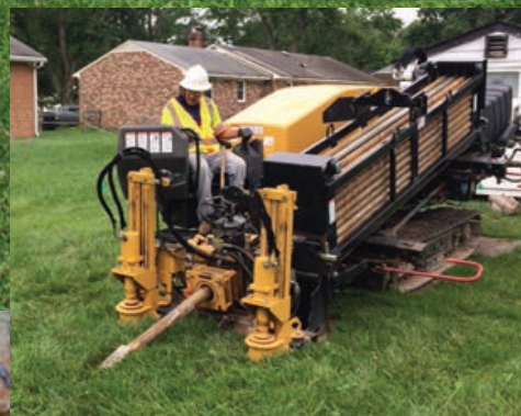
Dominion at work undergrounding transmission lines using boring.
