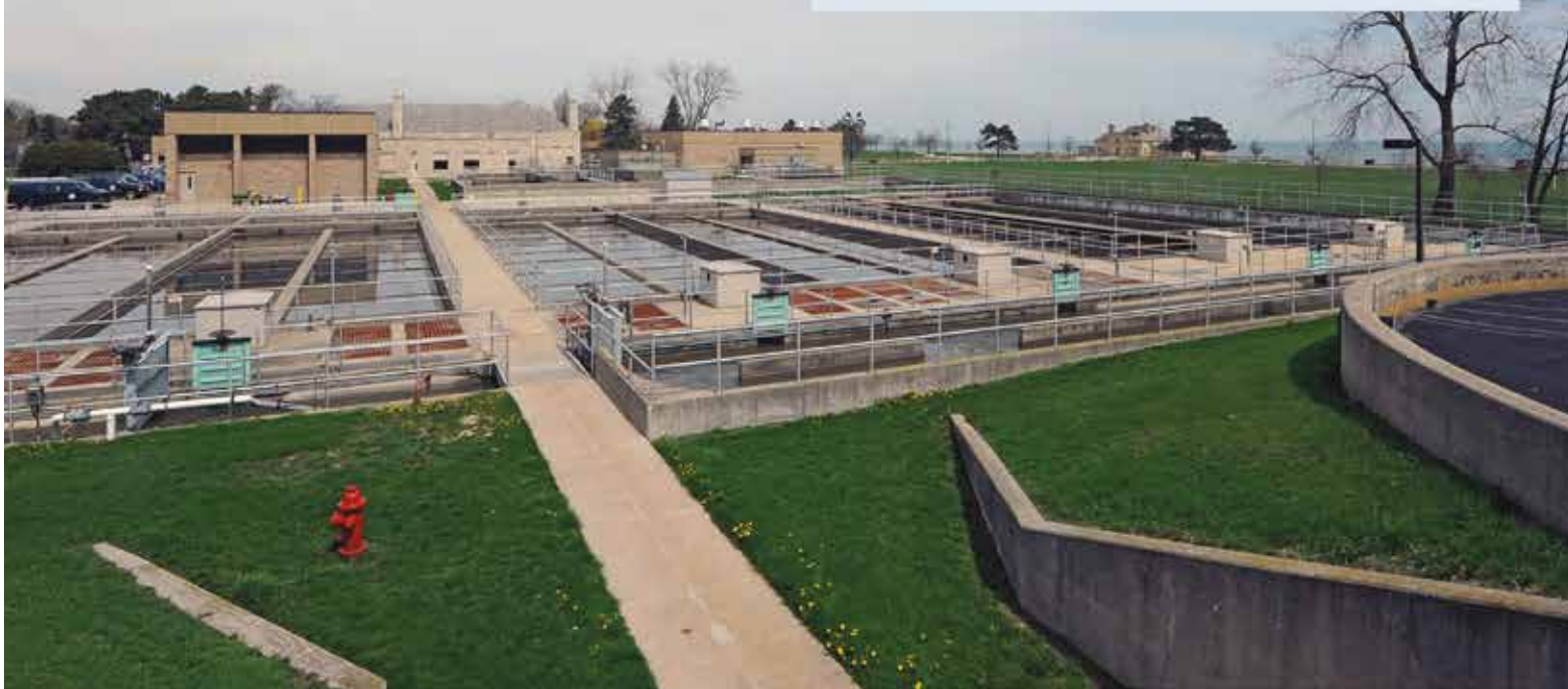
ABOVE: The Kenosha plant, on 29 acres along Lake Michigan, treats an average of 22 mgd and has a design capacity of 28 mgd. BELOW: The grit basins and primary clarifiers.
