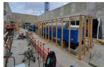
Metro Wastewater Reclamation District Denver, Colorado: Installation underway for MagPrex, a post-digestion P-recovery process and (8) SC26-4 dewatering centrifuges.
