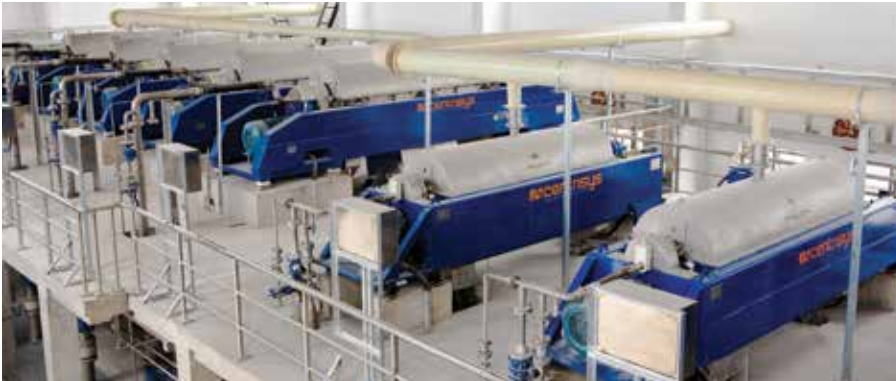
DingFuZhuang WWTP Beijing, China: Five Centrisys THK600 and four CS21-4HC.
