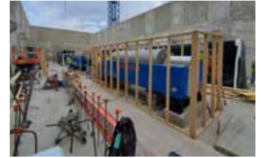
Metro Wastewater Reclamation District Denver, Colorado: Installation underway for MagPrex, a post-digestion P-recovery process and (8) SC26-4 dewatering centrifuges.
