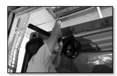
2.1.2. Fold at least 150cm of the TSL away from the door opening starting from the zipper. Then tape the folded section around the perimeter of the container door.
