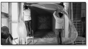
2.1.4. Place card boards on the TSL floor and along the walls for added protection;
