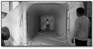
2.1.3. Secure excess liner material near the door perimeter by folding and sticking it on the sides of the door using tapes to prevent possible damage and to make it more accessible during loading.
