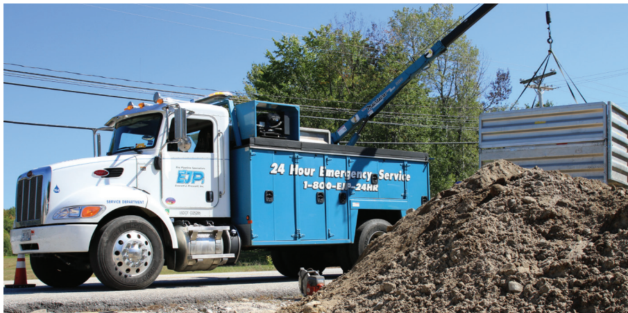
Team EJP Service Truck lowering trench box into trench.
