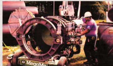
Former American Inland Marine's, Case Drott, holds Plexco HDPE pipe as EJP's Robbi Lockhart and retired EJP manager, Rod Dubois, prepare MegaMc machine that is welding pipe for Lake Auburn, ME, intake installation.
