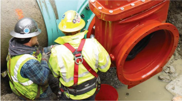
Team EJP's Service Department was recently on the job for Sappi to repair a problem with a 36" Pre-Stressed Concrete Cylinder Pipe. Sappi had noticed a leak beginning to surface on their critical raw water feed line, which feeds their entire property and production facility.
