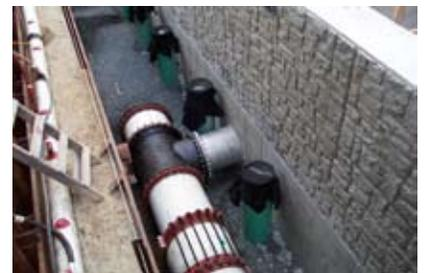
*Pictured are some of the epoxy coated 48" fittings at the intake structure. During high tide, river water flows through the 48" and 36" pipelines so it can be treated.*
