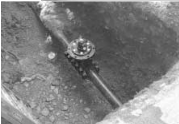
Photos above: Valve insertions for the village of Franklinville, NY. “Buffalo” Bob Gingerich is above right. Photo at right: Valve insertion for the town of Canadea, NY’s Waste Water Treatment Plant.
