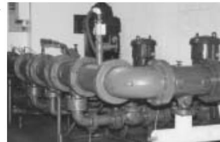
The existing steel pipe originally installed in 1993 was corroding and had started to form pinholes. EJP – Vernon contacted its sister company QWP and Jeff Carlos was sent to measure and lay out the project. The welded steel pipe with ductile iron flanged pipe and fittings were manufactured and shipped based on the dimensions he took at the site. The customer's comments say it all. *Great job, everyone.*
