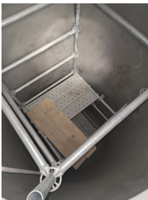
(Far Left) 100% containment achieved. (Near Left) A look inside the tank, post-blast, with suspended scaffolding. (Below) The exterior of the tank and entryway.
