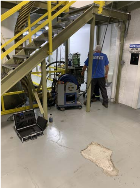
(Above Left) The heat curing equipment is set up to cure the ChemLINE® coating to spec. (Above Middle) The vent is set up to move the fumes out of the manufacturing facility. (Above Right) Heat cure equipment with an insulated vent extended from the heat curing equipment into the tank. (Bottom Right) Fully cured topcoat layer inside the storage tank.
