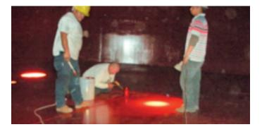
784-32 (gray) to the roof and walls and at 6-8 mils (150-200) microns wet film thickness in accordance to the specification.
