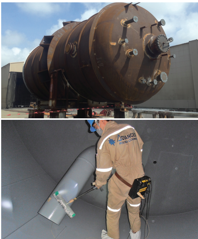
A new carbon steel vessel (top) is shown waiting for lining at KFPC in Taiwan. Spark testing of the finished ChemLine® topcoat (bottom) is done to prepare for storage of different proprietary polymers and specialty chemicals.
