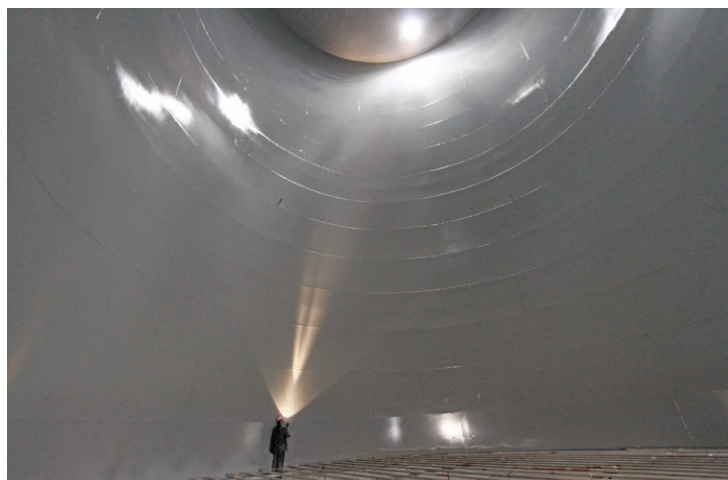
New tanks for Likit Kimya use ChemLine® 784/32 for Sulphuric Acid (red) and MEG storage (grey).
