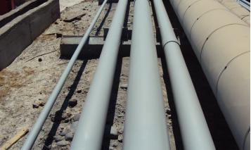
Various photographs show the external coating of ChemLine® 784/32 on these pipes at the Petkim refinery in Turkey. The base coat is shown in red, with the top coat in grey.
