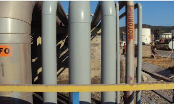
The ChemLine® base coat is shown in red, with the top coat in grey, on these pipes at the Petkim refinery in Turkey.
