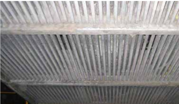
(Left) At this FGD system operation at a coal-fired power plant, flue gas attacks the alloy construction of reheat tubes after wet scrubbing. (Right) The reheat tubes
