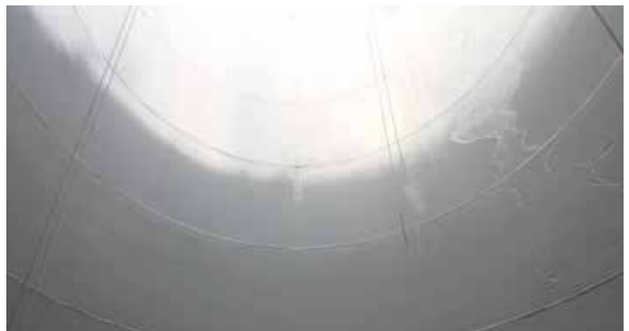
heat cured, covering an area of 20 meters high x 5-1/2 meters in diameter. After successful performance, the customer requested ChemLine® coating be applied to stack tunnels, condenser lines (sea water lines), process water tanks and concrete neutralization pits.
