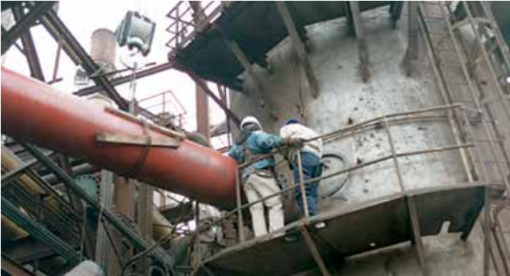
(Left) At this steel bar- and wire-producing facility, severe pipe and scrubber corrosion is caused by gas containing 5% Hydrogen, 5% Sulfuric Acid, and a slurry of iron dust, carbon and water, that travels through a 120-meter pipeline and empties into a large
