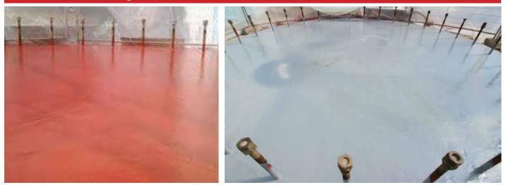
ChemLine® serves as a barrier on concrete surfaces, and for secondary containment against occasional splash/spill occurrences at facilities. LEFT: ChemLine® 784/32 red base coat applied on concrete surface. RIGHT: ChemLine® 784/32 grey top coat applied and then heat cured, serving as concrete and secondary containment protection against corrosive fertilizer chemicals.
