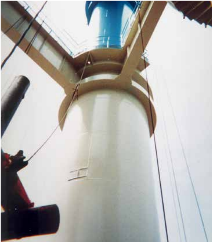
Closeup of coating on stack.
