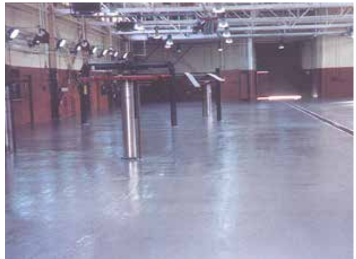
Vehicle maintenance area with ChemLine® coating.
