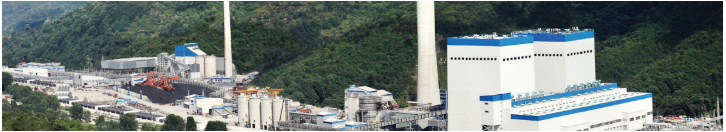
The Eren Energy (Eren Enerji) coal-fired plant in Turkey.
