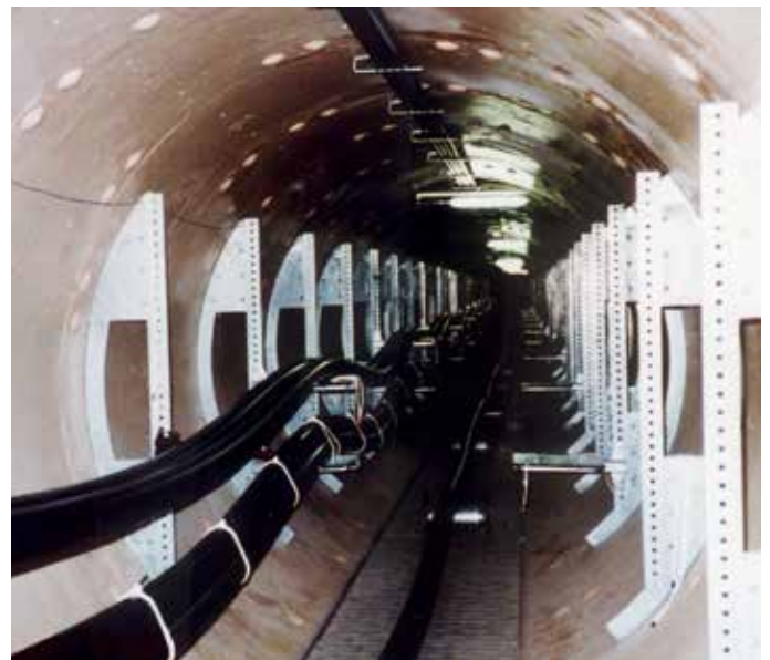
Tokyo Fire Department lines underground utility tunnels with ChemLine® for preventive protection.
