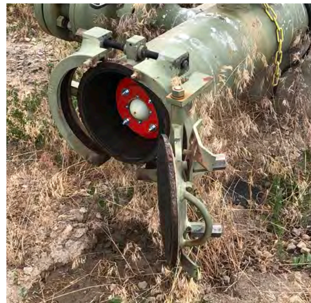
In gas pipelines, Pipers® are deployed through attachment to a cleaning pig.
