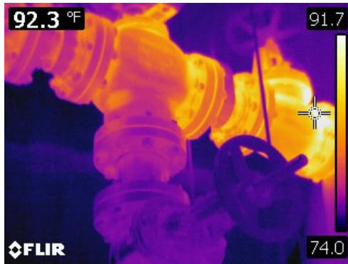
Bare heating valves in the Red Deer Provincial Building fan room.
