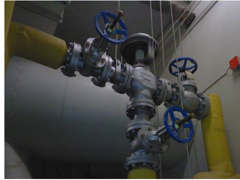
Bare heating valves in the Red Deer Provincial Building fan room.
