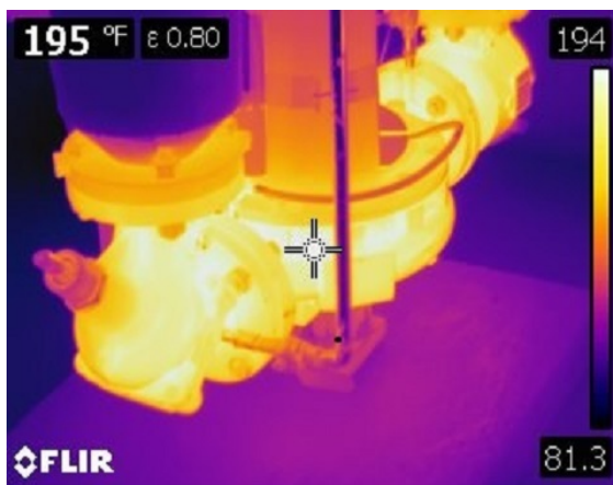
Bare heating pumps in the Boiler Room
