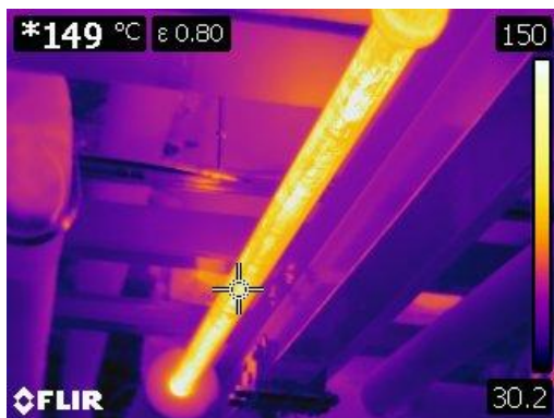
Figure 23 Thermographic image of a bare steam supply line at the entrance of the fan room.
