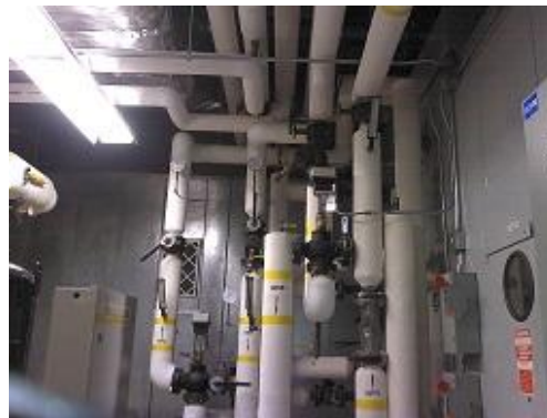
Figure 38 Conventional image of the same lines to unit. Bare three way mixing valves and control valves.
