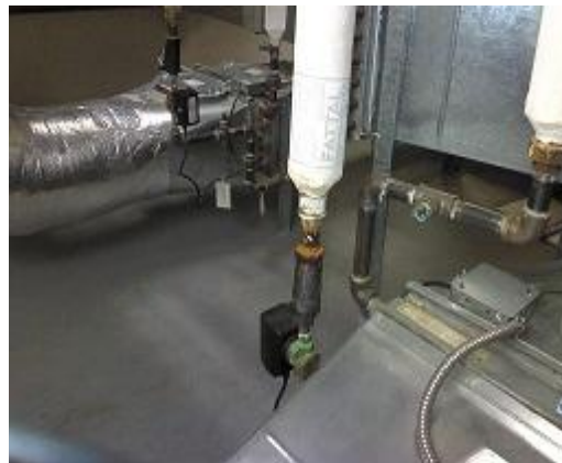
Figure 48 Conventional image of the same iron heating lines to the coils.
