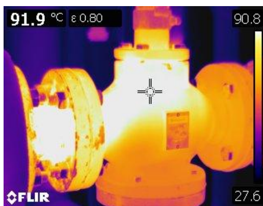
Figure 51 Thermographic image of three way mixing valve.
