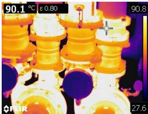
Figure 55 Thermographic image of exposed heating pumps and associated piping.
