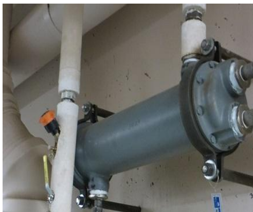
Figure 18 conventional image of a similar heat exchanger.
