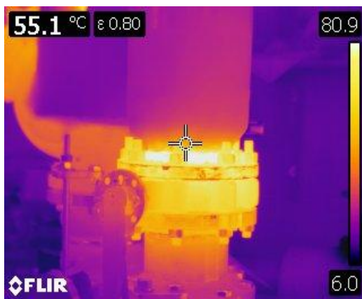
Figure 9 This is a thermographic image of the supply lines to a circulation pump on the hot water system. The lines and the pump should be insulated to conserve energy.
