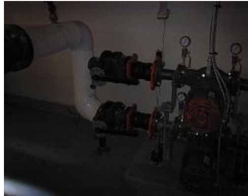
Figure 54 Conventional image of exposed heating supply lines to pumps.
