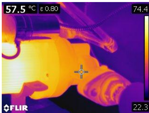
Figure 43 Thermographic image of exposed heating pump.
