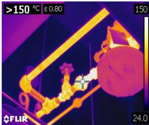
Figure 7 This is a thermographic image of bare by-pass piping and associated valves and strainers.
