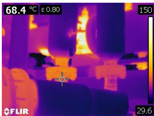
Figure 29 Thermographic image of heat exchangers and pipe flanges to heat exchangers.
