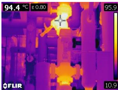
Figure 37 Thermographic image of heating supply lines to unit.
