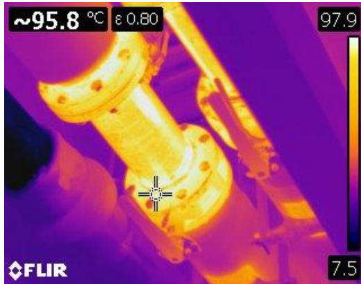
Figure 21 Thermographic image of bare steam lines above the entrance of the fan room.
