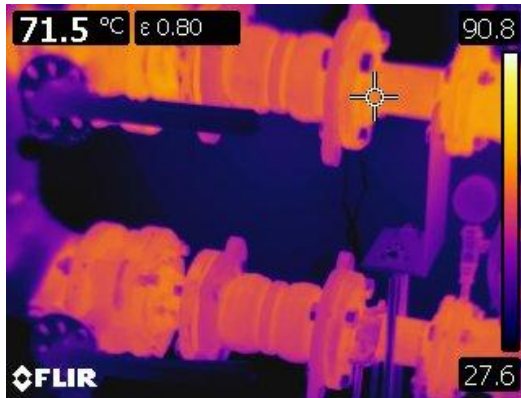
Figure 53 Thermographic image of exposed heating supply to pumps.
