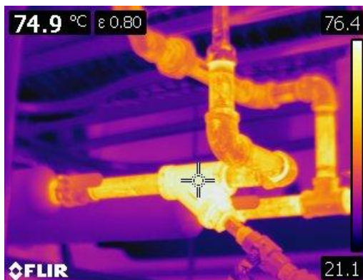
Figure 43 Thermographic image of exposed heating pump.
