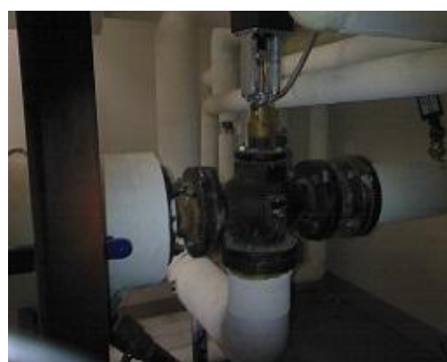
Figure 52 Conventional image of the same three way mixing valve.
