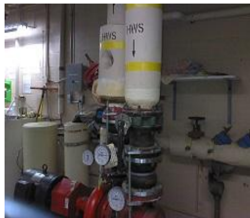
Figure 10 This is the conventional image of the supply and return lines at the back of the boiler.
